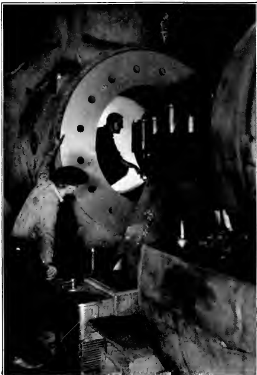
BORING A LARGE CYLINDER IN HAMILTON MACHINE SHOP
